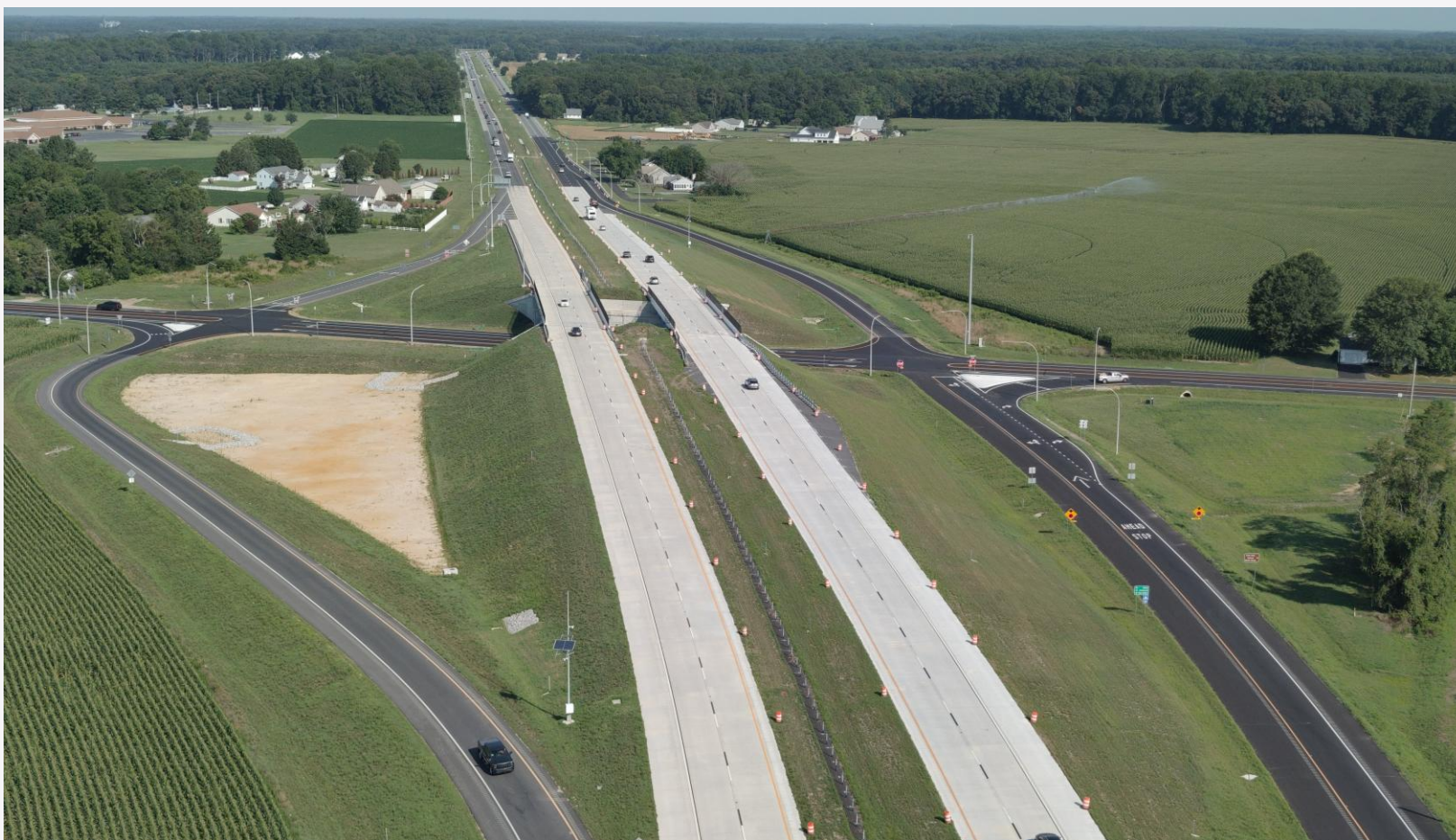
State Route 1 over State Route 16 in Sussex County
