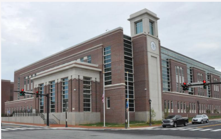
New Kent County Family Courthouse, Dover
