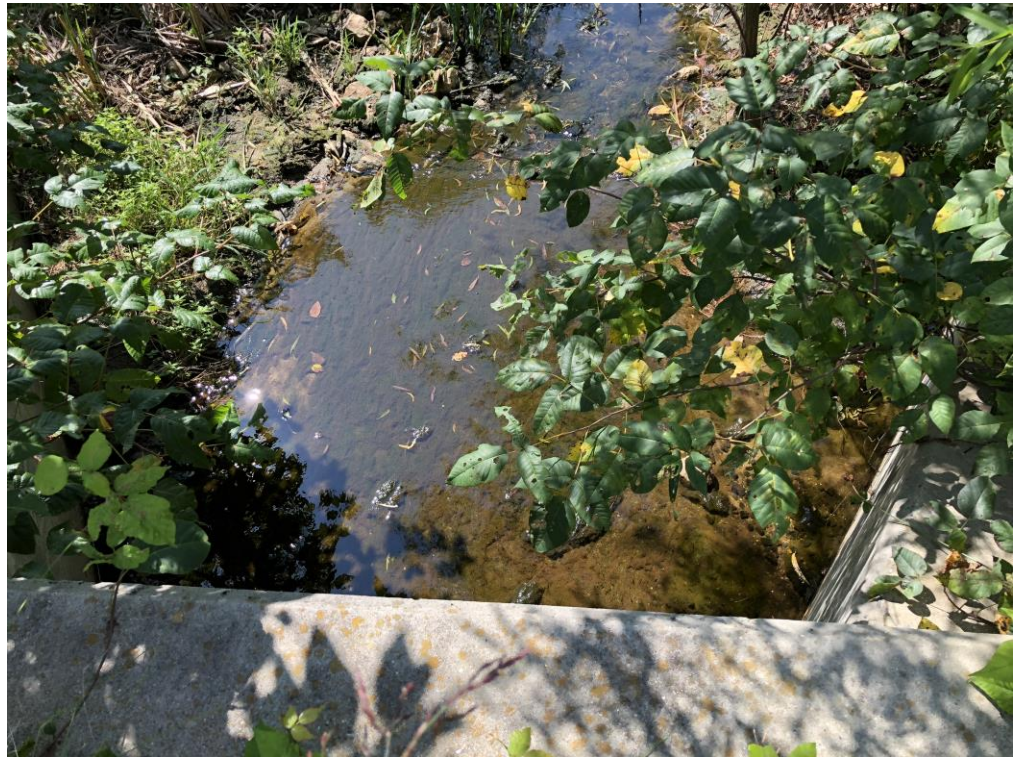
Photo 2: Outlet from Pond
