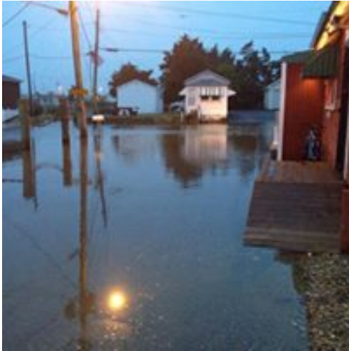
Example of flood event in front of the Bayview Inn on Murderkill Avenue
