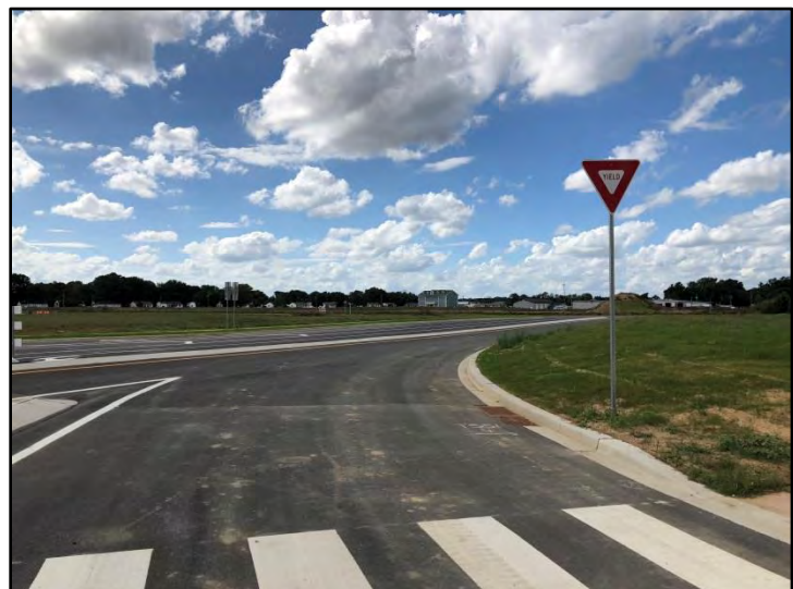
Future Camden Bypass off Route 13
