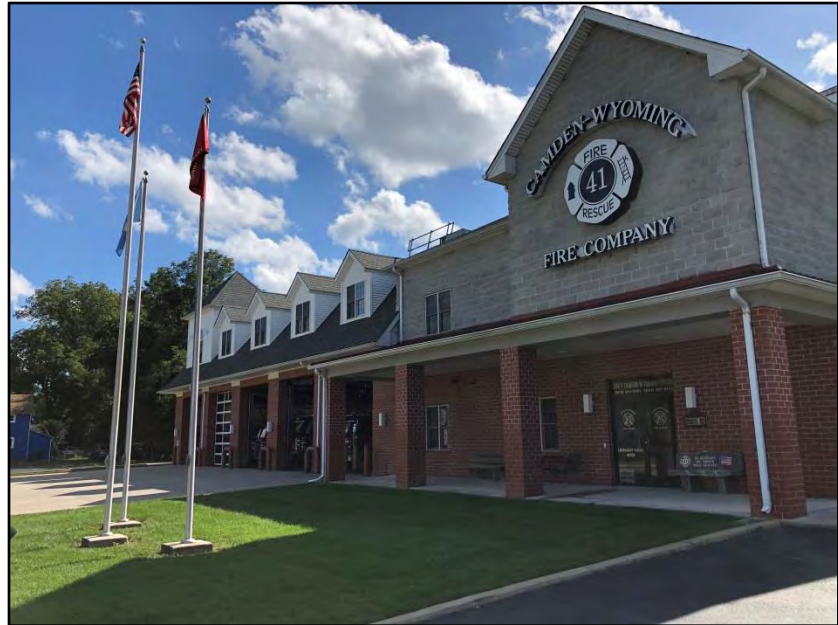
Camden-Wyoming Fire Company headquarters
