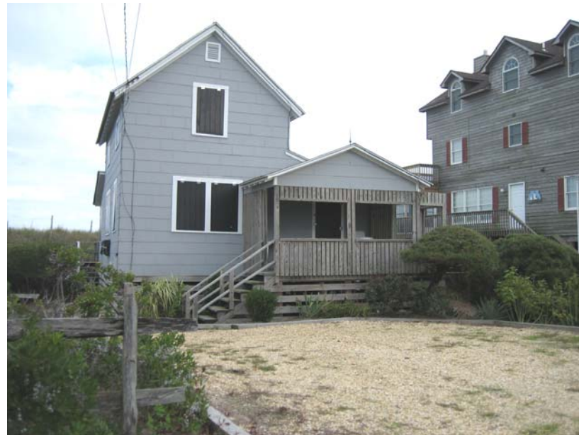
An original cottage.
