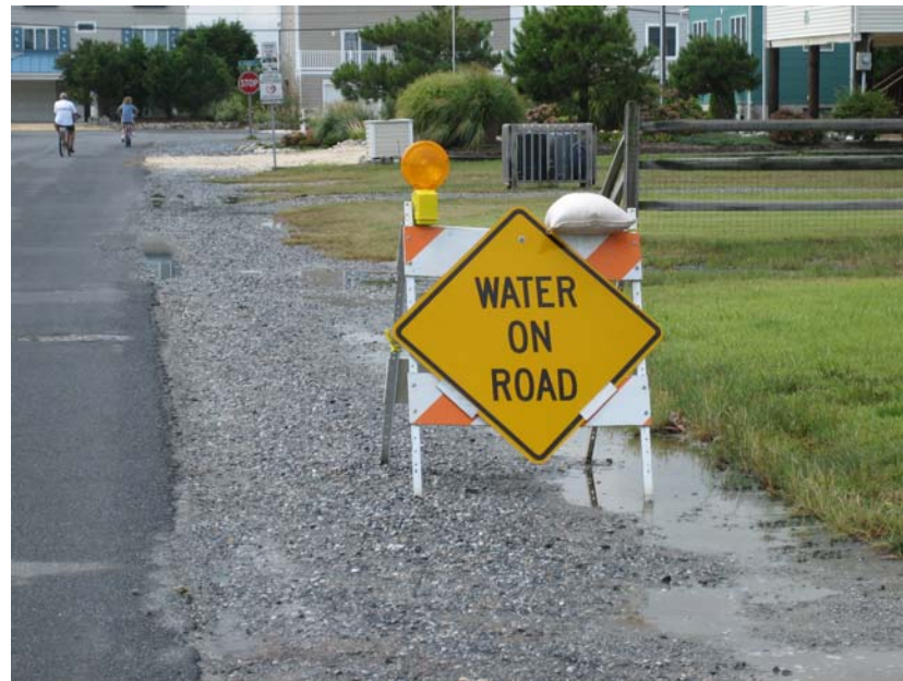
The Town's Five-Year Road Damage Improvement Plan addresses drainage concerns.
