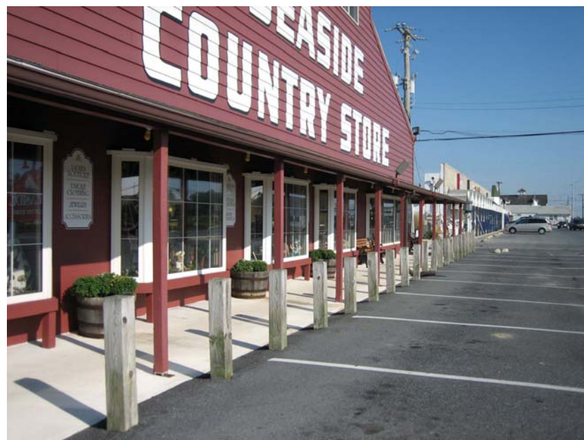
The Seaside Country Store is an example of iconic architectural character.
