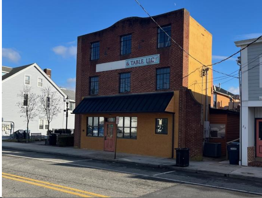
19 W. Commerce Street – Circa 1890 three-story commercial building most recently utilized as a sit-down restaurant on the 1 st floor. The current owner partially renovated the building in 2017 and utilized DDD grant rebate funds. Upper floors have been vacant for many years while 1 st floor restaurant space has been vacant since 2023.
