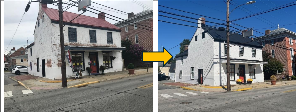
Before and after photographs of exterior façade improvements to the Yarn Maven at 62 W. Commerce Street which also included the construction of a new 2 nd floor 1-bedroom apartment dwelling unit.
