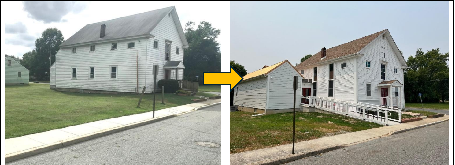
Before and after photos of renovations to Mt Olive Pentecostal Church at 139 N. East Street
