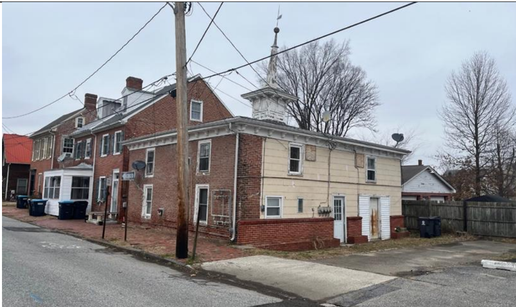
10 N. Delaware Street – Circa 1860 former carriage house for the former Clement's Mansion at 56 W. Commerce Street which was converted to three residential apartments in the mid-20 th century. The building has remained vacant for a number of years, and was recently purchased by a local contractor who plans on renovating the building to construct modern apartment units.
