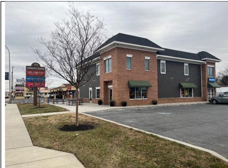
New two-story mixed-use building constructed in 2018 with 1 st floor ice cream store and 2 nd floor computer support business along U.S. Route 13 at the edge of Smyrna's DDD.
